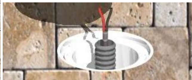
Carry out the electrical connection paying attention to the cables polarity and fix the lighting body with 2 screws
