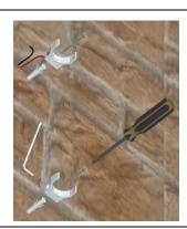
Fix the brackets with screws suitable to the support.
