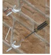
Fix the brackets with screw suitable to the support
