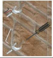
Fix the brackets with screw suitable to the support
