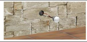
Carry out the electrical connection and insert the lighting body into the formwork
