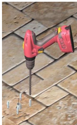
Drill holes for the screws compartment
