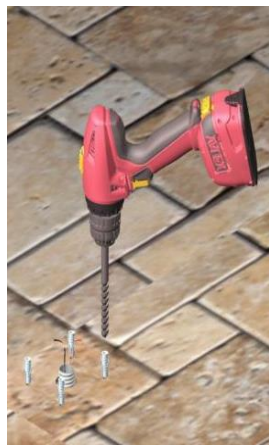
Drill holes for the screws compartment
