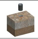
In the floor, insert and glue with silicone the formwork
