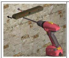
Positioning the support and carry out the hole for fixing
